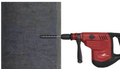
Step1 - Hole Drilling
